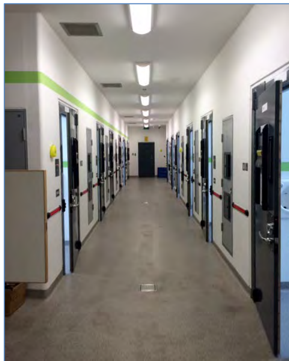
Figure 1: View of a Custody cell corridor
