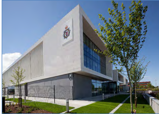
Figure 9: Bridgwater Police Centre. Far right ground floor is the Custody Unit
