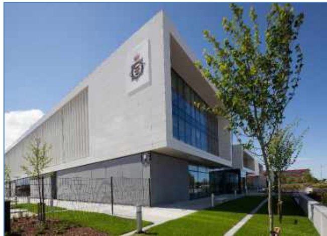
Figure 7: Bridgwater Police Centre. Far right ground floor is the Custody Unit
