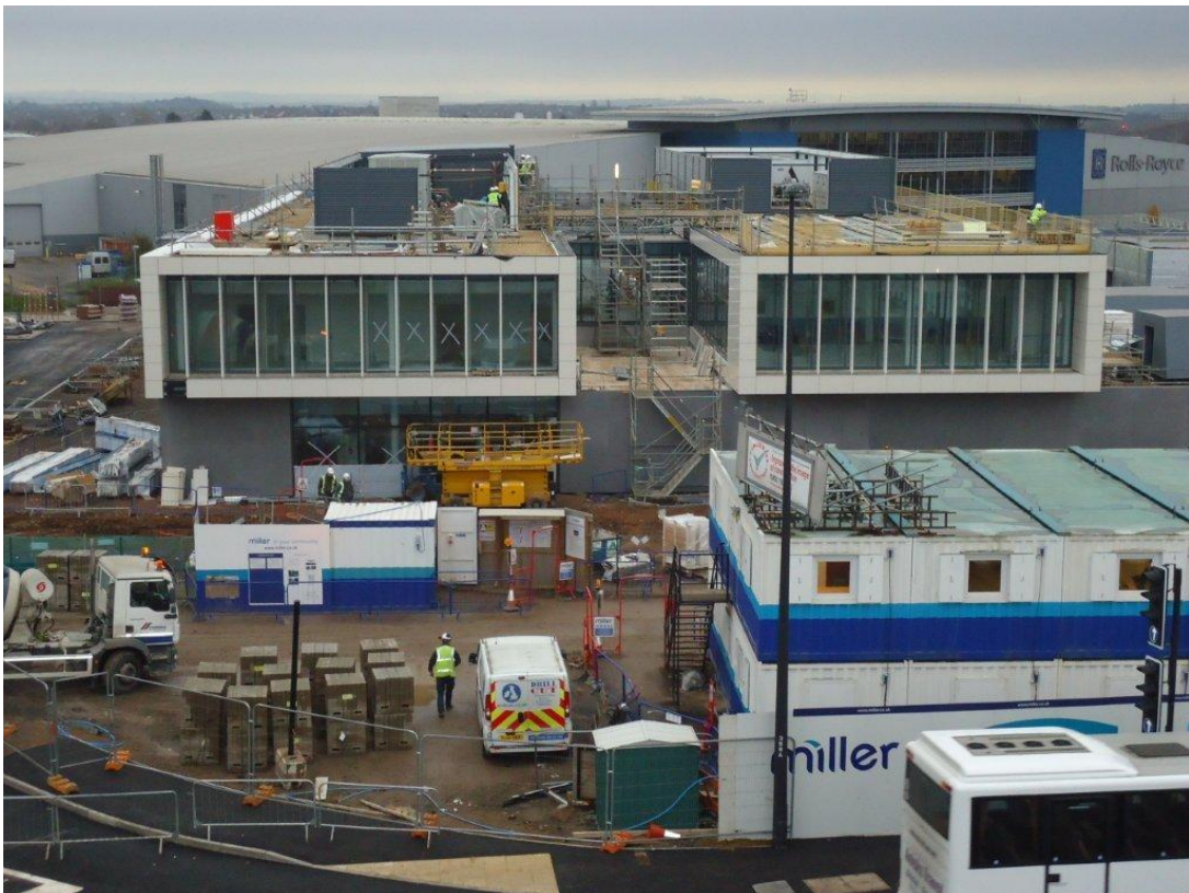
Gloucester Road, Filton – in construction
